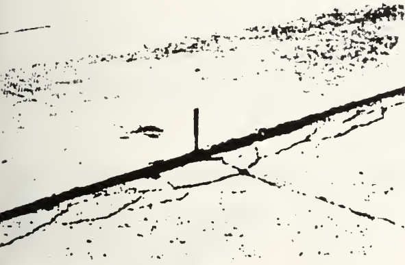
Fig. 3.2.3.8 — Lane/shoulder dropoff
